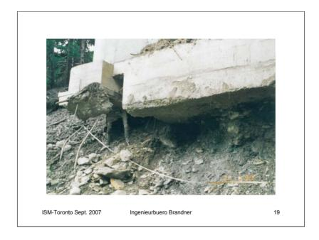
Damage after slide of slope in spring 1999 – micro-piles fully without any damage
