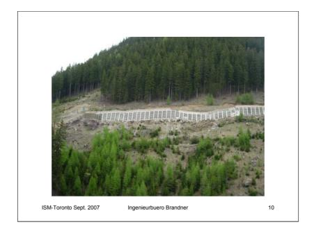
A 2-3 m thick layer of moraine gravel above a rock surface parallel to slope. The new erected ski run and road to the top of the mountain had to be reconstructed after one year in charge. This picture shows the situation at beginning of May.
