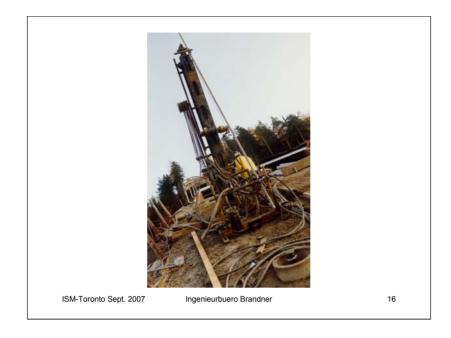
Reconstruction of a ski jump slope – the concrete slab had to be supported and doweling against slide – lightweight drilling equipement
