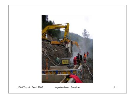
Reconstruction with pile foundation – IBO R51N bearing and tie piles length up to 8 m.
