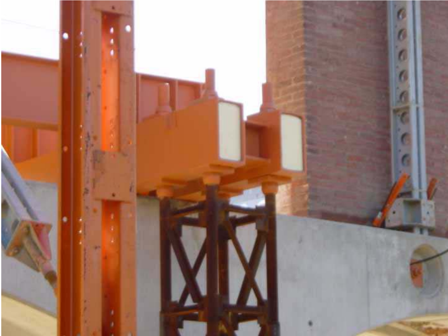
Details of temporary support.
