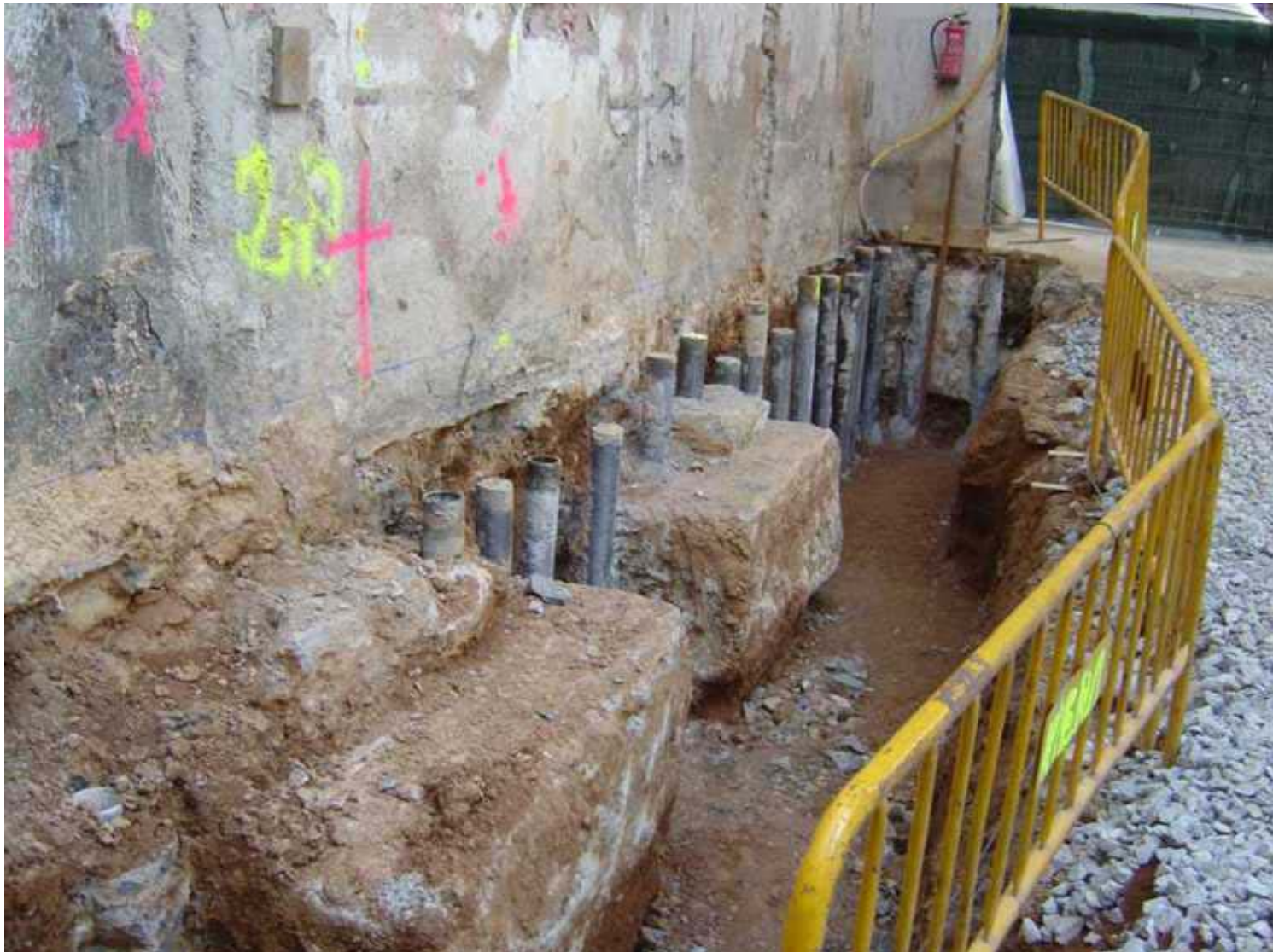
Existing Foundations or obstacles are penetrated by the micropiles.
