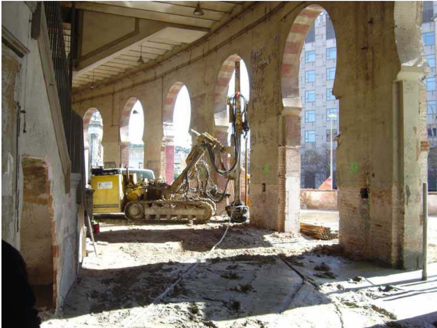
Difficult Access for Drilling and Grouting the Micropiles.
