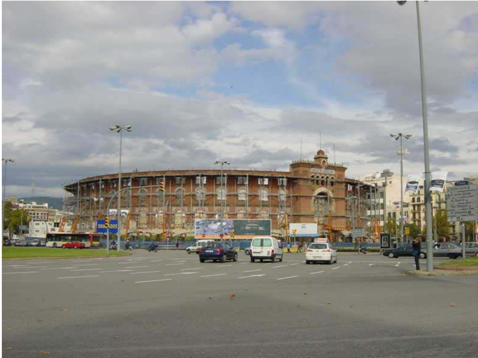
Still Existing Facade of Bullring
