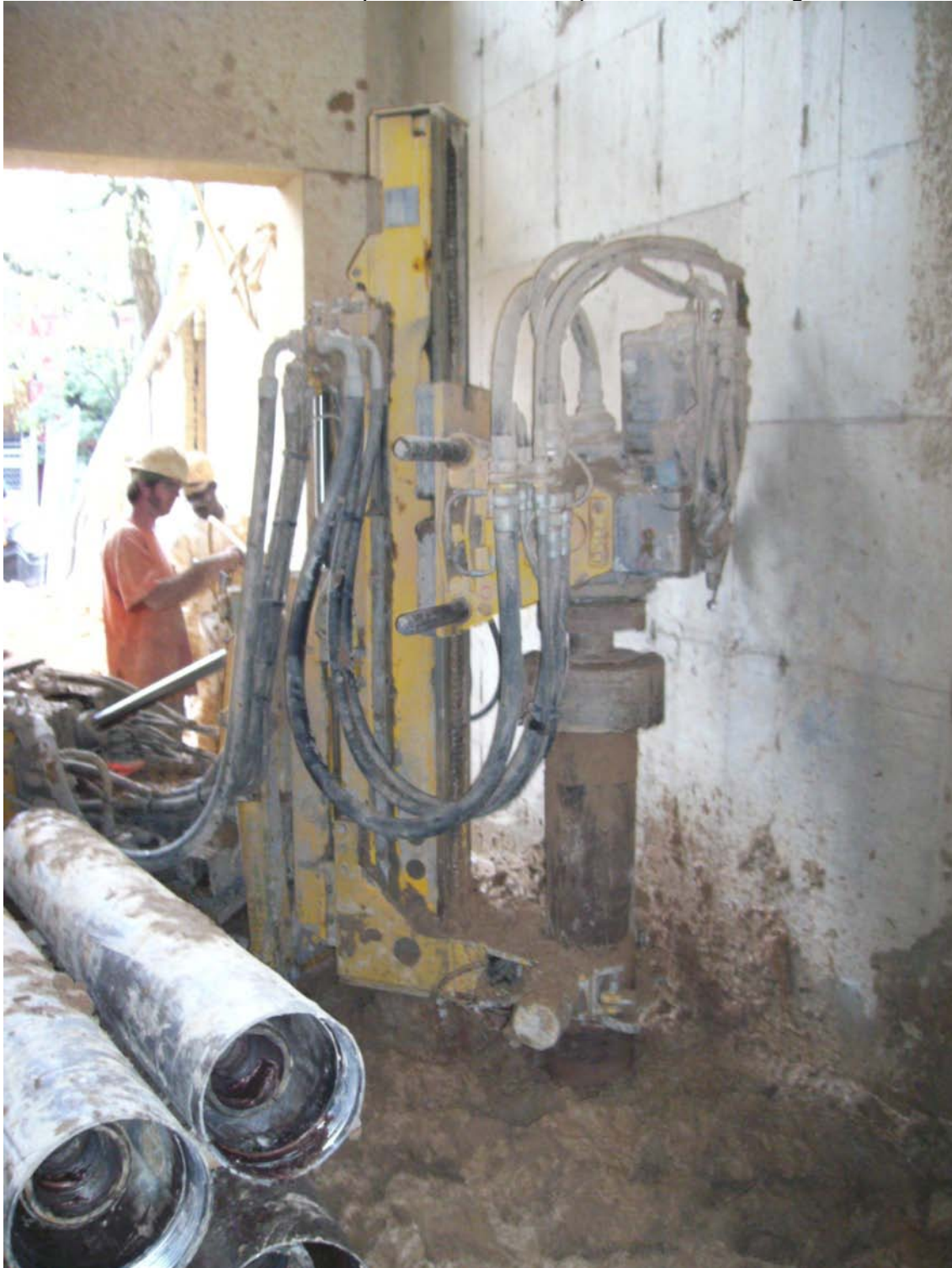
Figure 4 Micropile Drilling Operation
