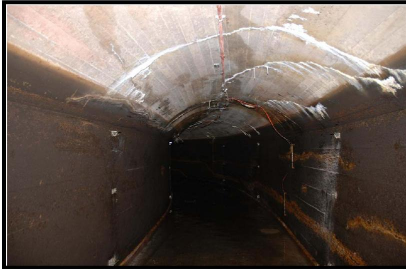
Figure 4: Photograph taken inside of the conduit showing spiral cracking
