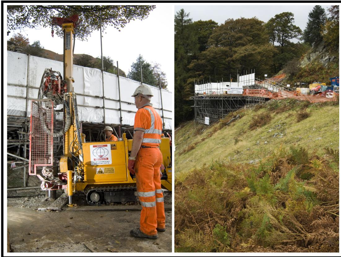
Figure 6. Light-weight drilling operating of temporary scaffold platform
