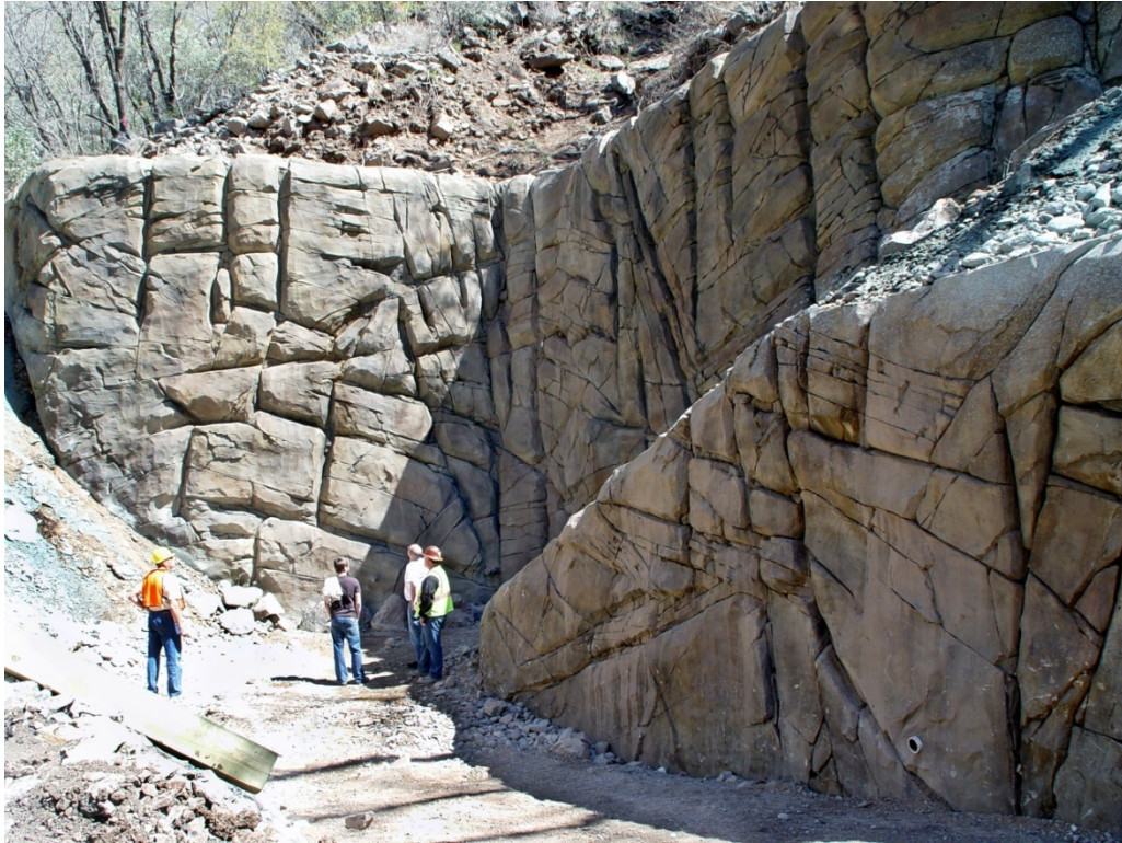
Photo 5 – Completed North Basin
