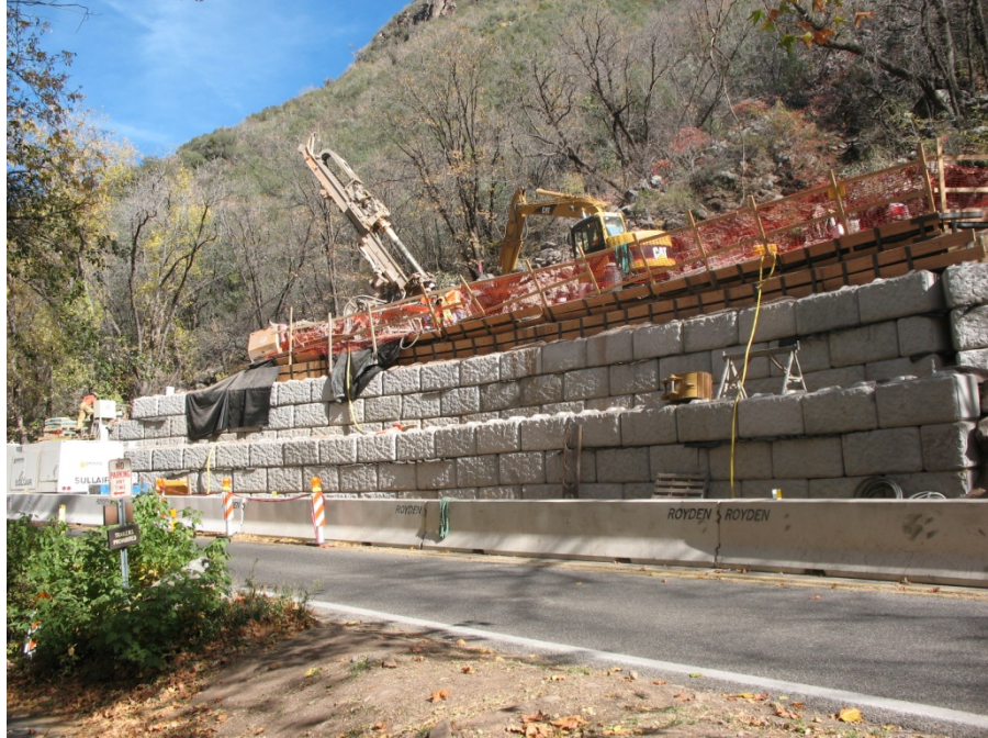
Photo 3 – North Wall Access Bench
