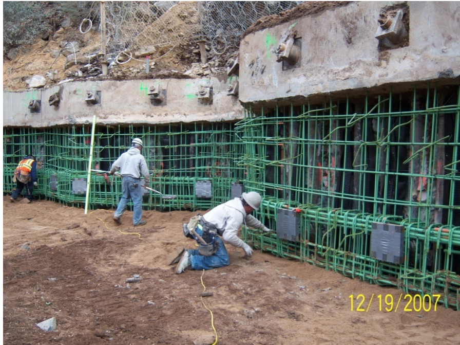
Photo 4 – Shotcrete Fascia @ Anchor Row 2
