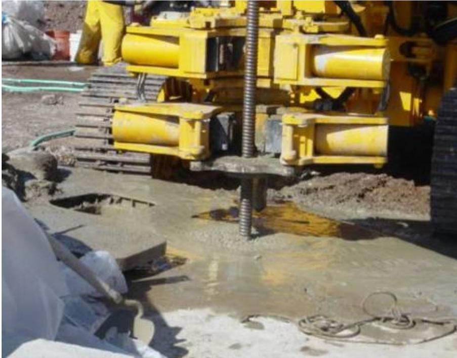
Figure 26, Observing Grout Outflow
