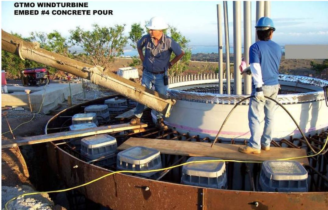
Figure 24, Casting of Pile Cap
