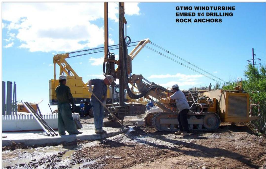
Figure 25, Drilling of Hollow Core Micro Piles
