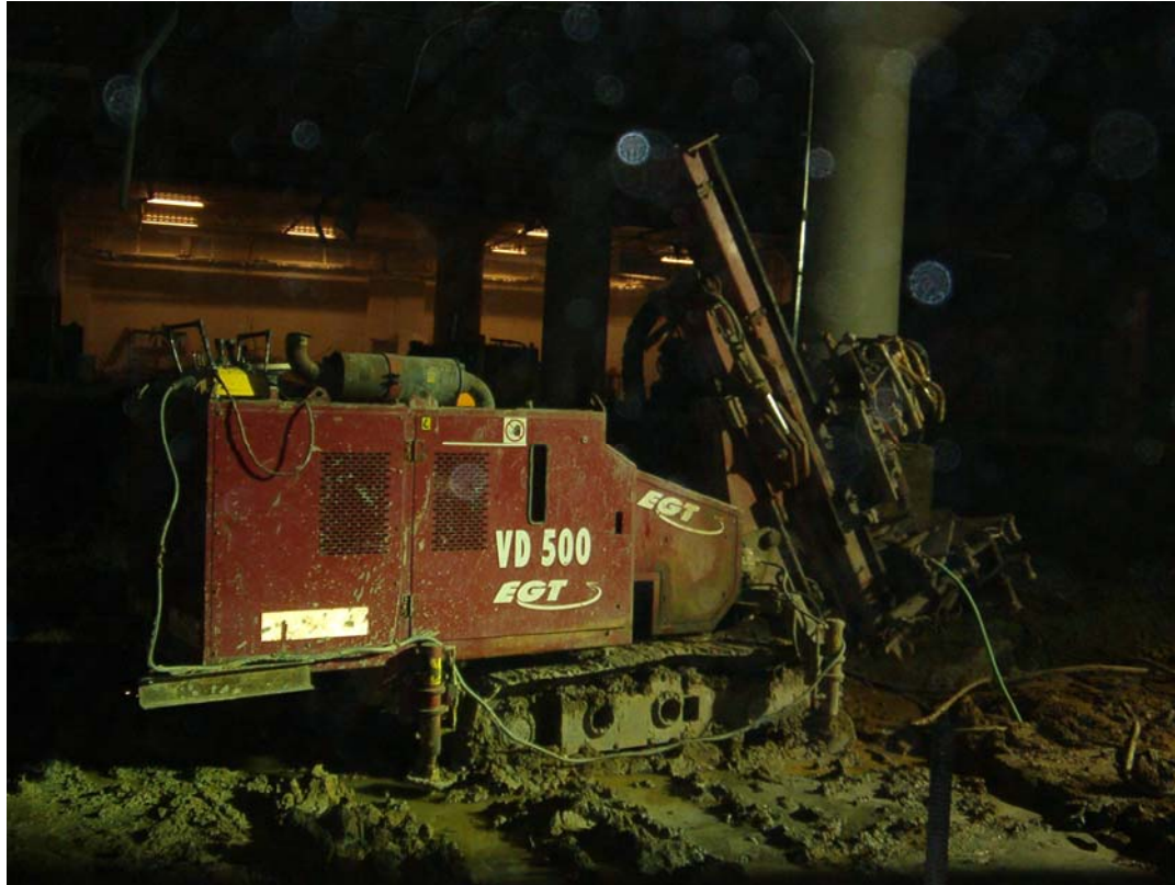
Fig. 8. Low Headroom Installation of Titan Micropiles at One NoMa Station.
