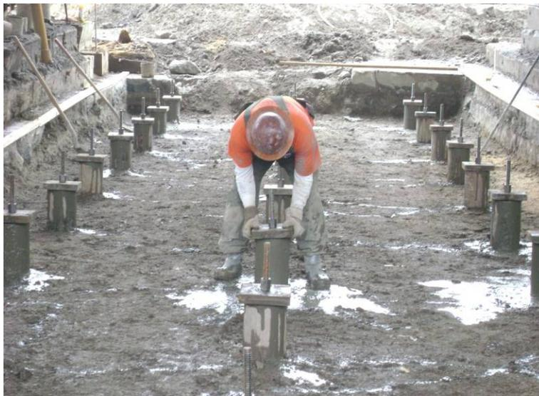
**Figure 8. Cutoff micropiles with pile-top connections installed at Pier 10S**
