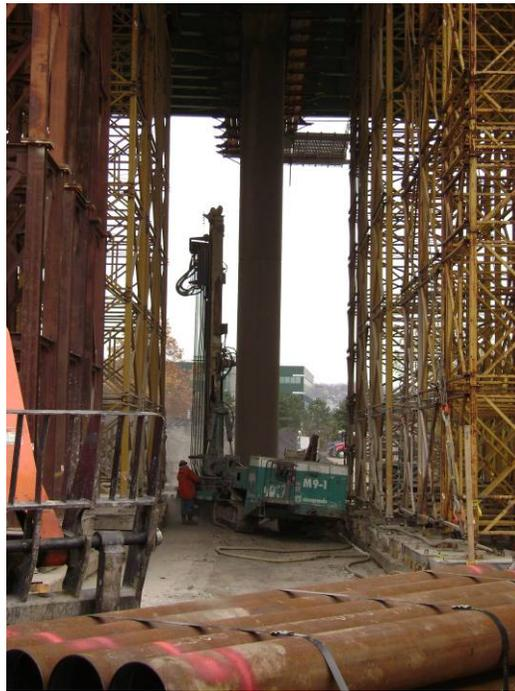
**Figure 7. Casagrande M9-1 hydraulic drilling rig operating within 4.9 wide area at Pier 10S**
