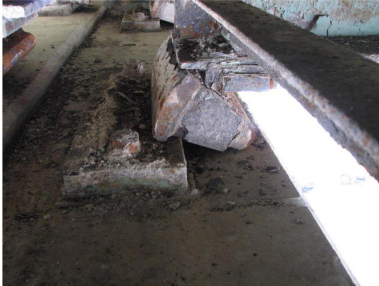
**Figure 1. Failed rocker bearing at Pier 10S (adapted from Splitstone et al, 2010)**
