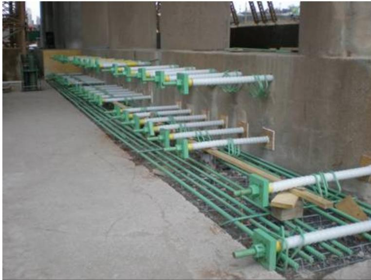
**Figure 9. Post-tensioned pile cap (adapted from Splitstone et al, 2010)**
