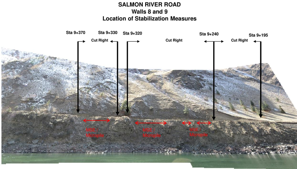
Figure 1 –Left shift of alignment (toward outside shoulder) with micropile MSE wall stabilization areas.
