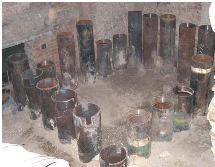
Figure 2. A pile group during construction at Cannon Place
