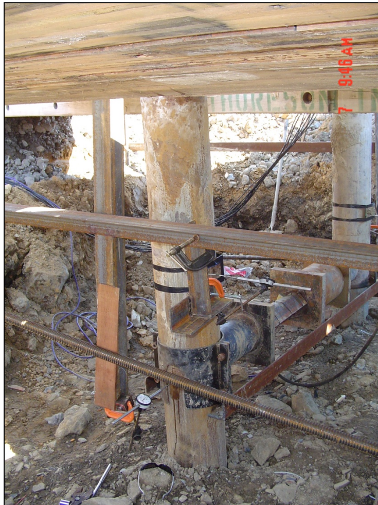
Figure 3 – Lateral Load Setup
