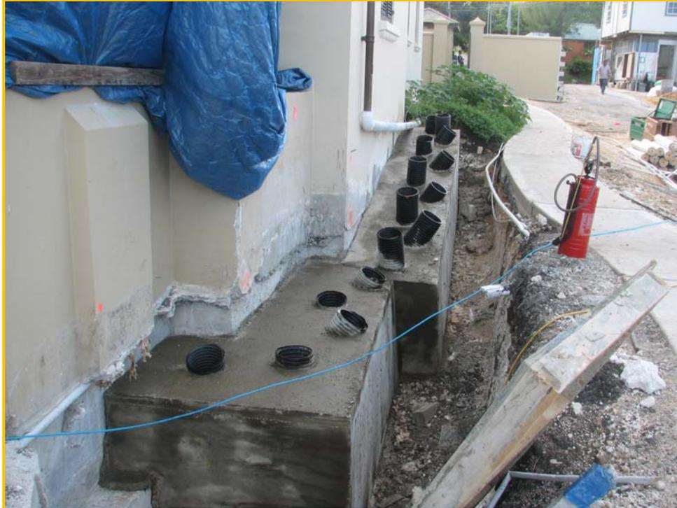
**Figure 9: New Grade Beam around Foundation**
