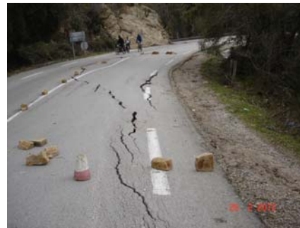
Photo 2: Landslide: pre-failure
