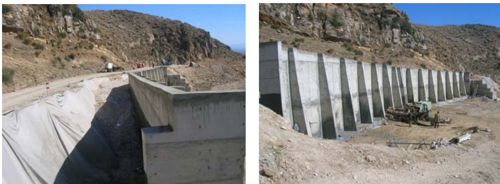
Photos. 2. Anchors works in progress
