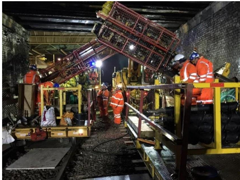
Figure 3: Drilling with Cages Confined Access – Keller UK
