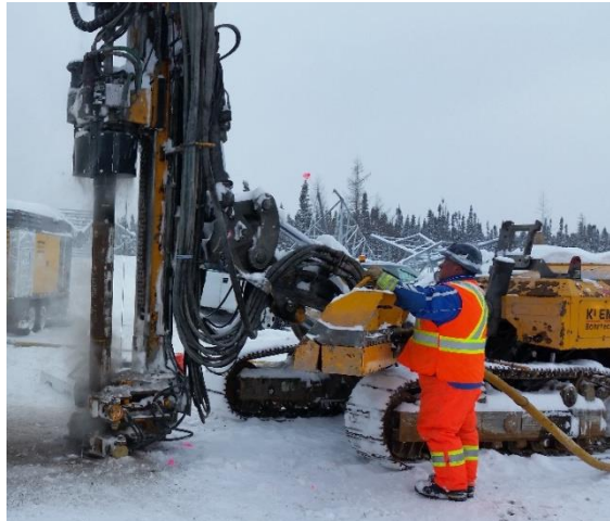
Figure 9. Micropile installation
