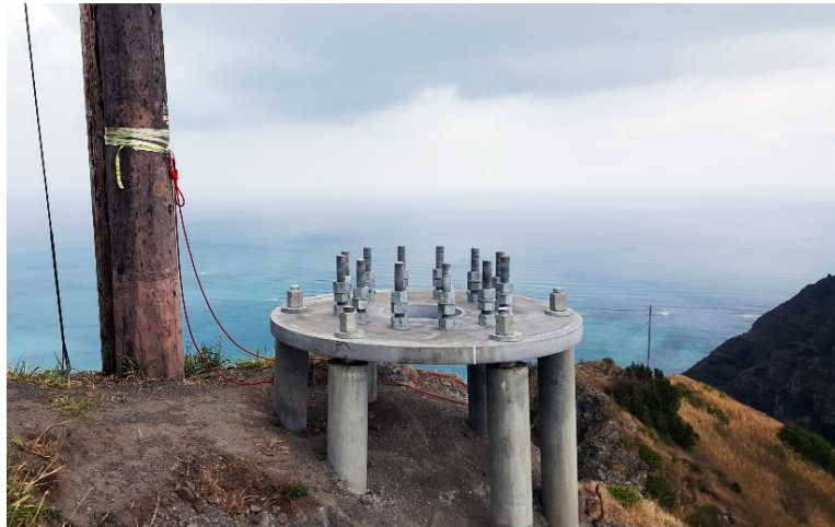
Figure 5. Completed steel cap micropile foundation
