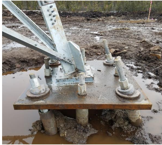
Figure 11. Installed D2/E1 steel cap micropile foundation
