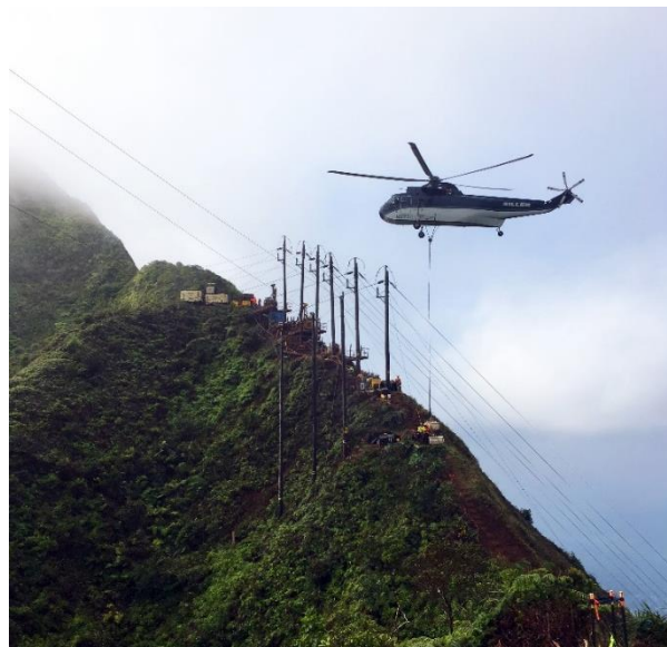
Figure 1. Replacement structures on steep ridgeline
