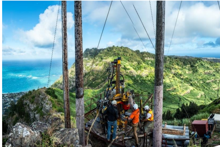
Figure 4. Micropile drill setup
