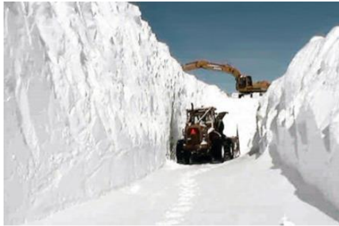
Figure 6. Example of ice road cut through deep snow
